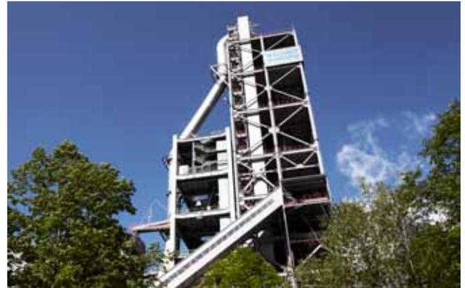
Anhovo upgraded their traditional suspension preheater kiln into a modern In-Line Calciner (ILC) Preheater system, chosen for its good performance with all fuels.
