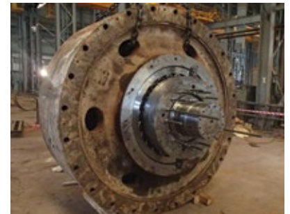
Replacement of bearing and grinding roller
