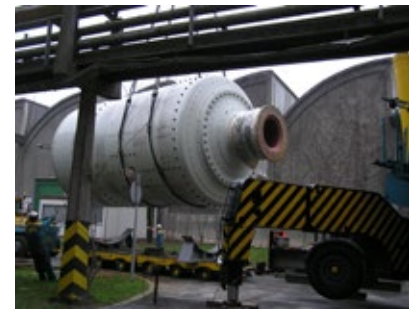
Replacement of ball mill shell with trunnion
