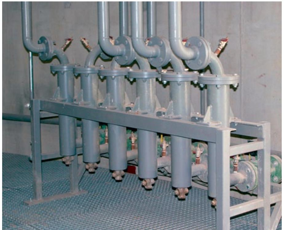
Figure 6: Filter battery for a single sector (optional)
