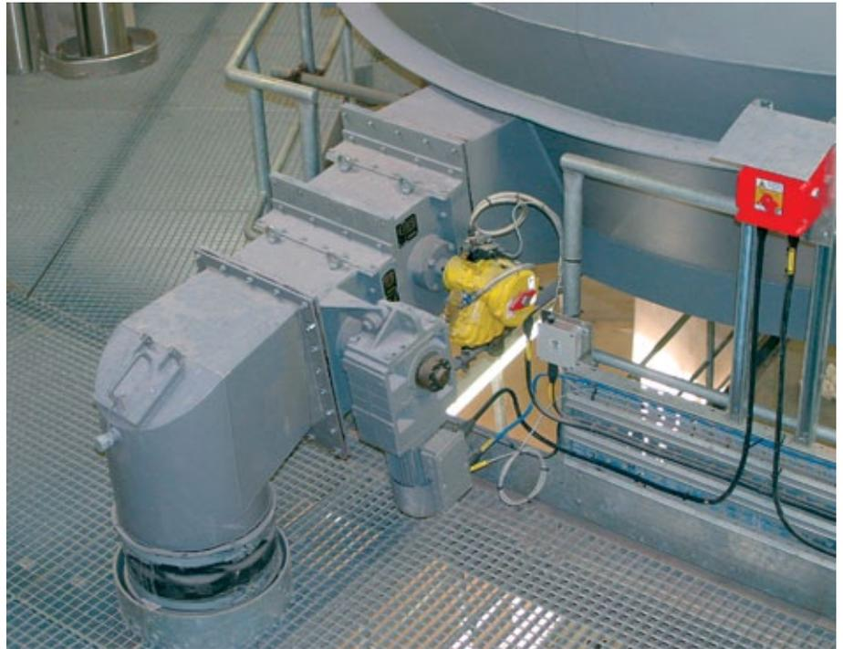
Figure 5: LOW kiln feed tank outlet
