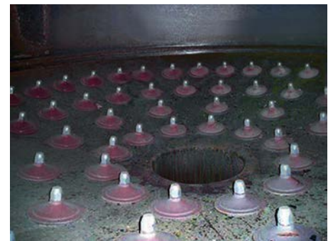
Fluidized bottom using Fullerator aeration/vibration pad
